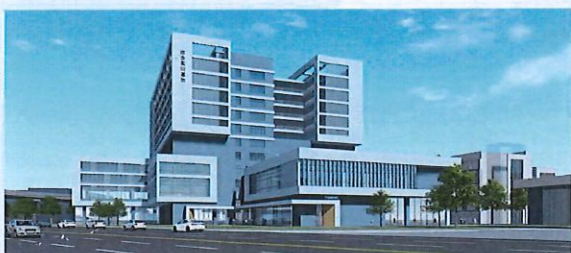
(在建实训大楼)
